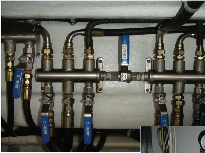
Left, steering manifold with bypass valve labeled. Below, a steering oil reservoir equipped with an air pressure gauge and oil level windows.
