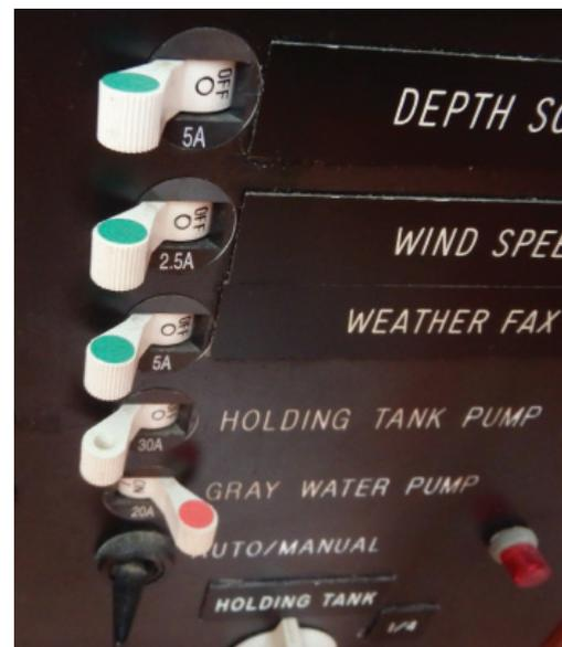
These circuit breaker switches are set up to accept color-coding indicators so that breakers can be set up in functional groups.
