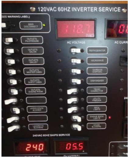
An AC electrical panel with both a voltage meter and an amp meter and separate sections for 120- and 240-volt circuits.
