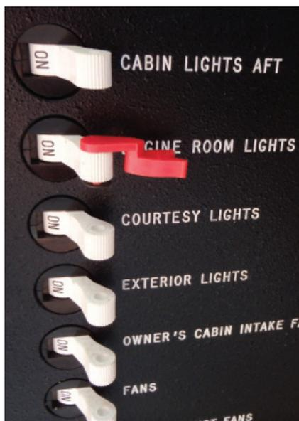
This shows a breaker reminder identifier. This is a visual and tactile way to remember to shut off or turn on a needed circuit.
