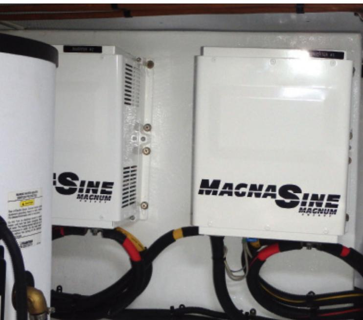
Two inverter/chargers side by side in an engine room. This setting provides easy access and good protection for the units.
