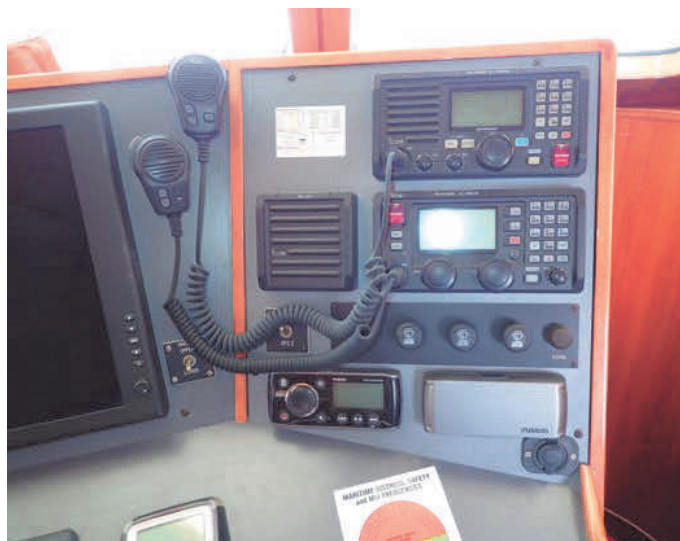
Two built-in VHF units with distress frequency buttons and a label with distress frequency intro.
