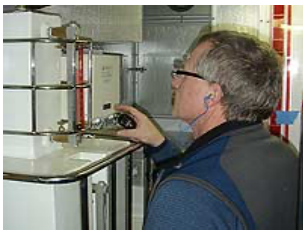
Brandy in engine room
